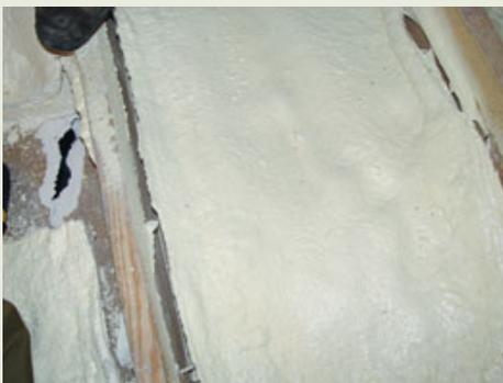
◀ Closed-cell foam was sprayed too thickly into this stud bay and has shrunk away from the framing as a result of exothermic heat build-up. The foam should be removed and replaced.
