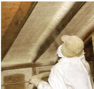
Open-cell foam can be installed in a single pass (above left), but because of its high expansion rate it must typically be trimmed after installation, which produces considerable waste (above). Trimming usually isn't necessary with closed-cell foam, but to avoid excessive exothermic heat, it should be installed in lifts no more than 1½ inches thick (left).
