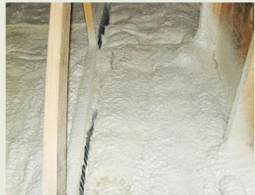
▲ This foam has pulled away from the truss chord due to excessive exothermic heat. Closed-cell foam should be installed in lifts that measure less than 2 inches thick, and with enough time between lifts to allow exothermic heat to dissipate.
